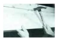
3. Hook bottom lip of track cover onto mounting bracket, nail top in place above track plank.
