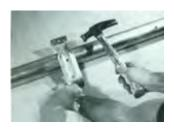
Tap shoulder rivets on mounting brackets into slotted key-holes on the track.
