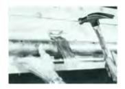
2. Now nail mounting brackets to track plank with ordinary ring shank nails. No lag-bolts needed.
